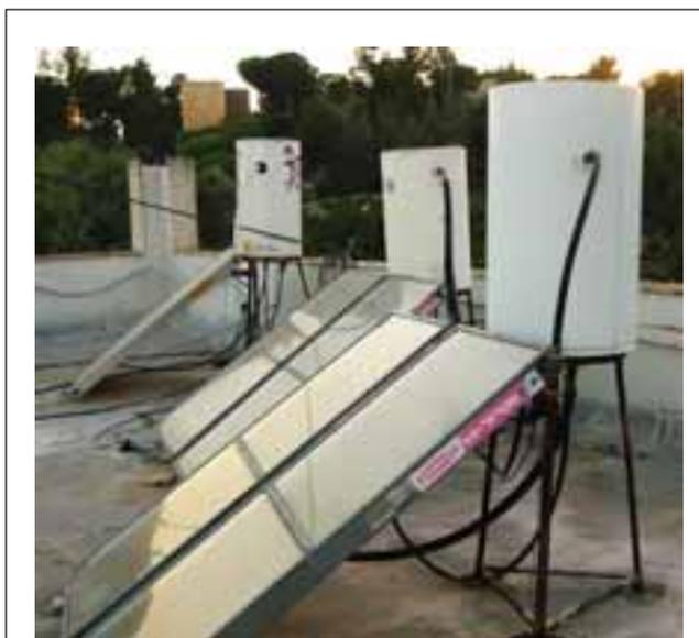
**Figure 2** Flat plate solar water heaters on residential rooftops<sup>3</sup>
